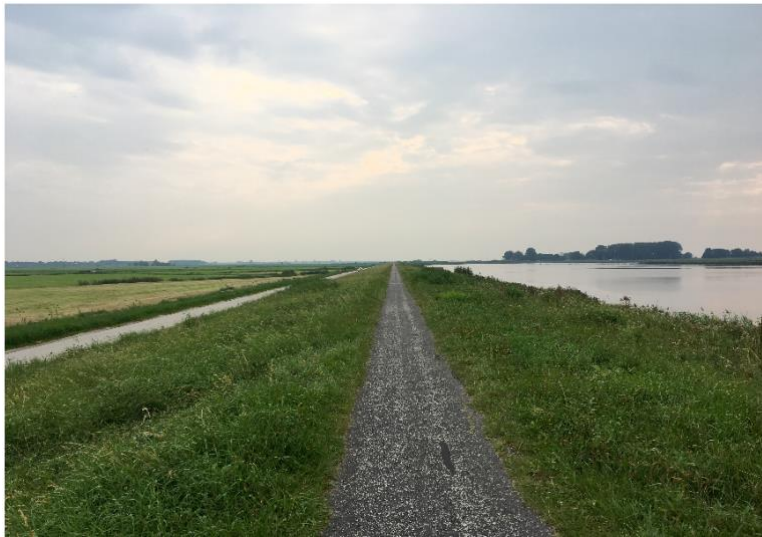
Figure 5. A dike near the town of Putten in the Netherlands, where the recent EGU-sponsored “Nethermod” meeting was held in late August 2017. This dike is one of many in the Netherlands that protect negative-elevation land (left) from a higher sea level (right).
